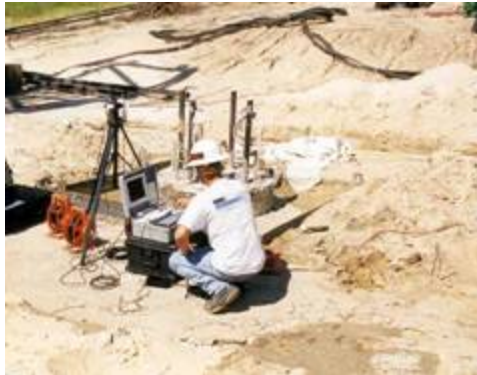
CSL Test in Progress
