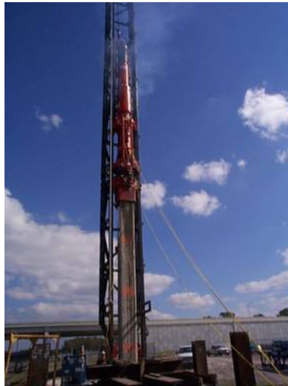
Pile driving with impact hammer
