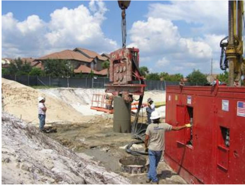
Drilled Shaft casing extraction with vibratory hammer.
