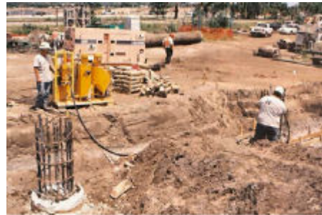
Post Grouting of Production Shafts
