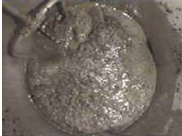
View of shaft bottom through Mini-SID camera with 2.5 inches of sediment
